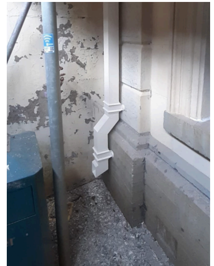
Guttering and downpipes fitted.
