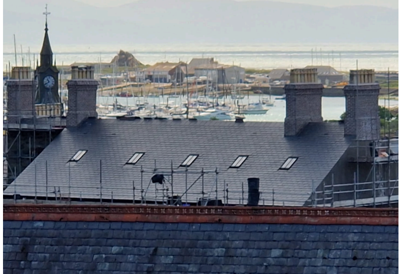
The new roof is looking good.
