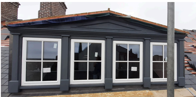
Dormer windows completed
