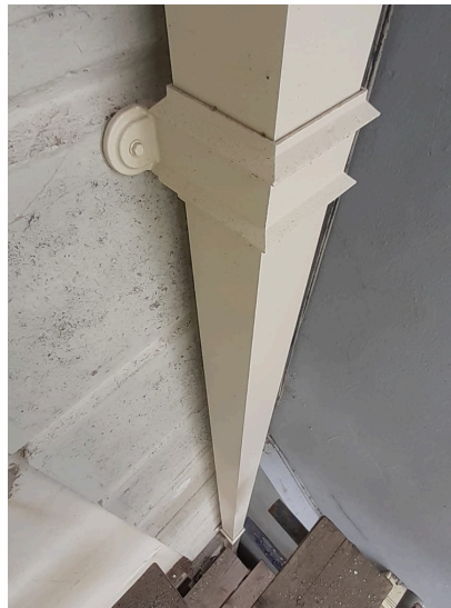
Guttering and downpipes fitted.
