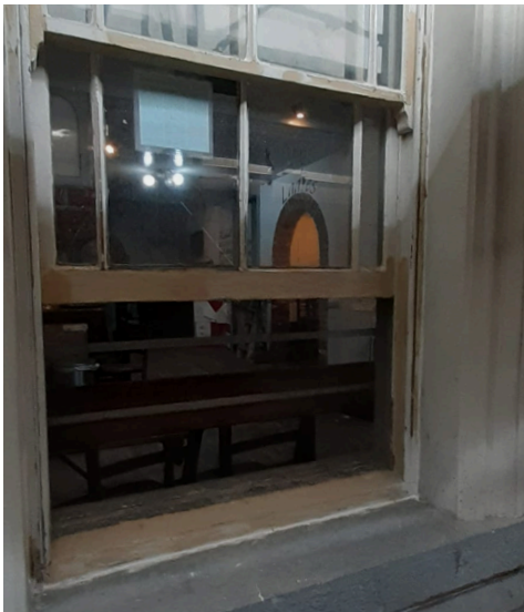
Renovated windows ready for paint.
