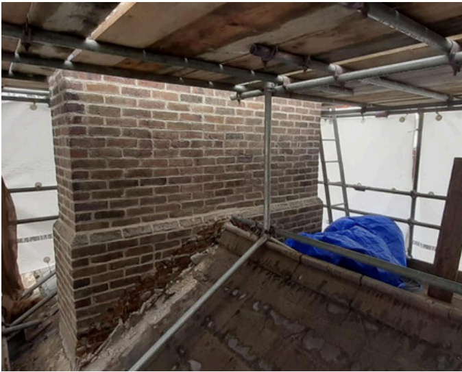
The repointing of the chimneys has been completed
