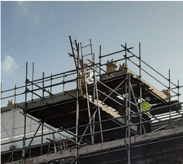
Removal of chimney from rear of building
