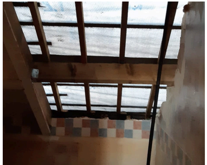
Dormer windows removed from the rear of the building.
