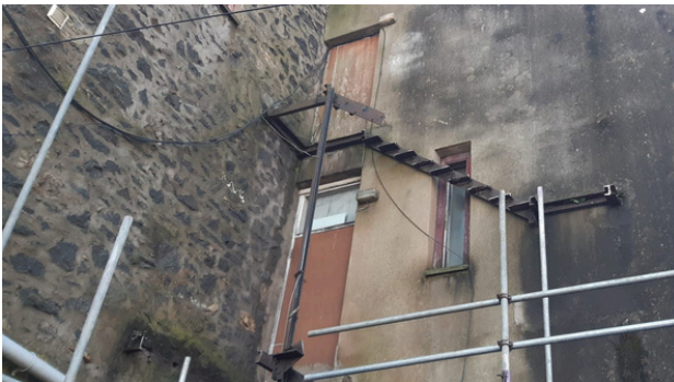
The dangerous fire escape has been removed
