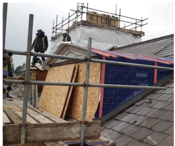
Renovation of the dormer windows at the front of the building
