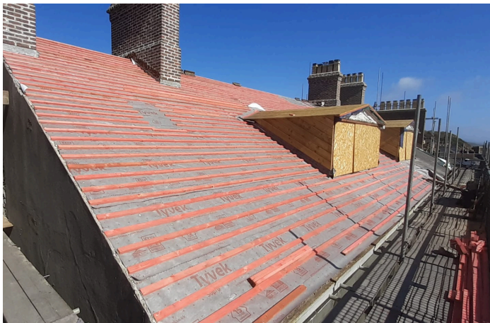
Finished batten work at the front of the building
