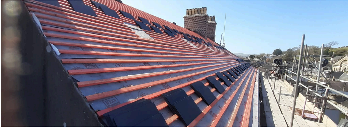
The new roof ready for the slates to be installed.
